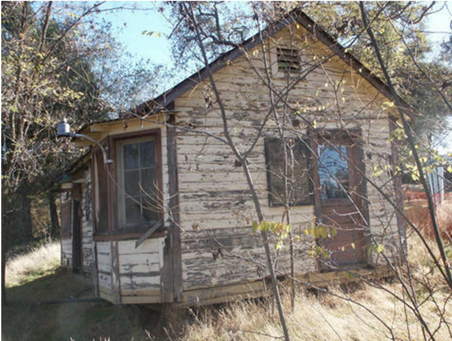
Notice more weather effects towards bottom of building. Peeling paint.
